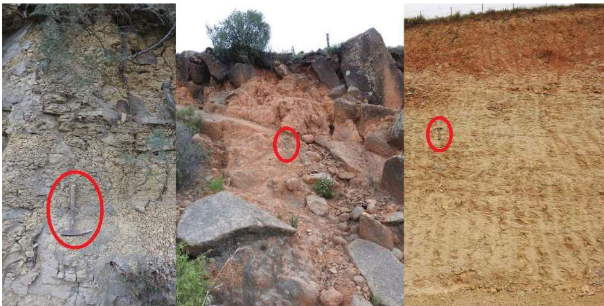
Figure 3.7. Depth of the weathering zone in soils in the KwaZulu-Natal midlands, geological hammer for scale (Van Tol and Van Zijl, 2022).
